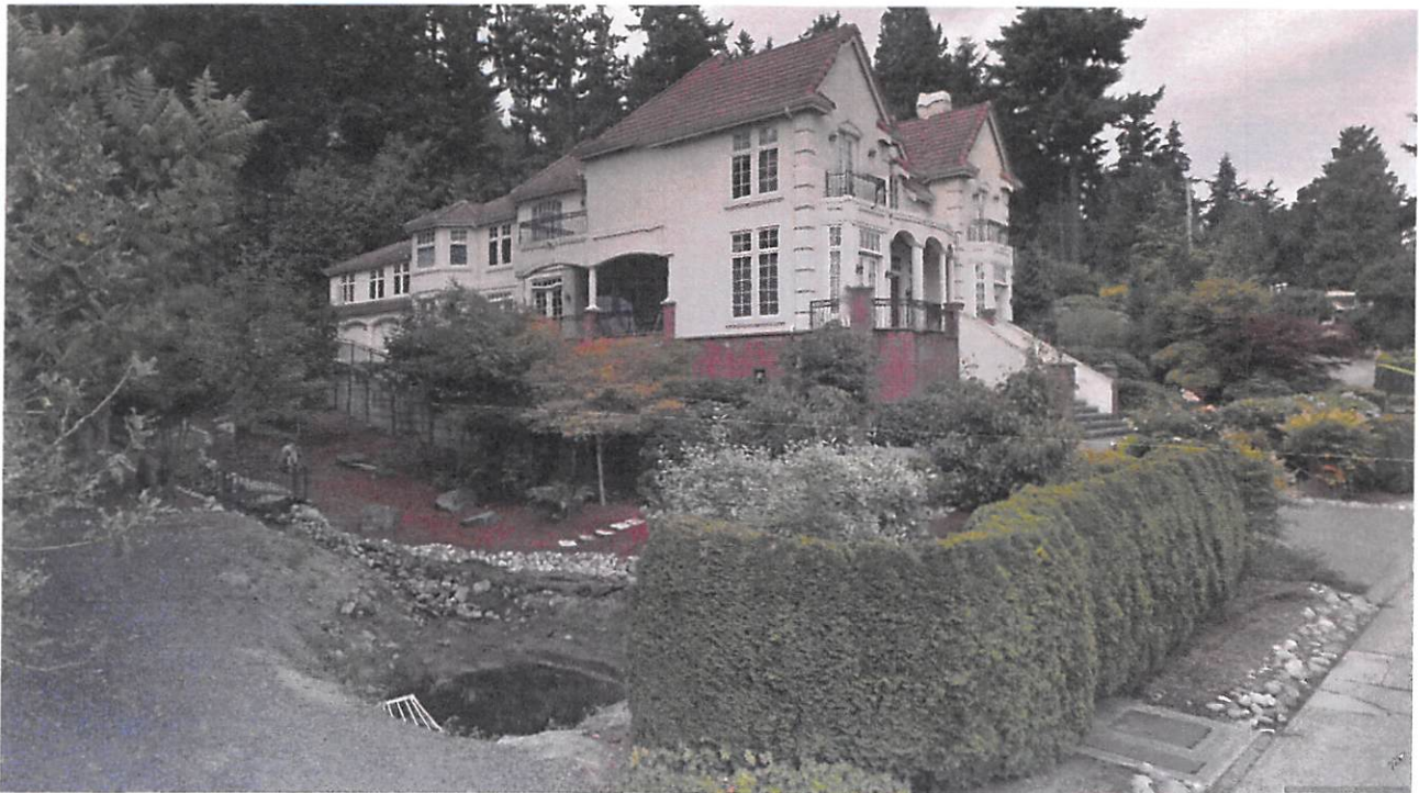
The Glenhome Sediment Pond
